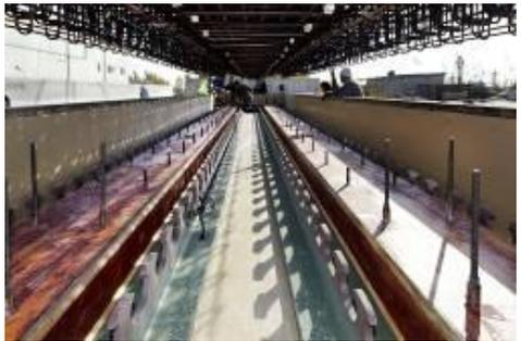
Figure 14 - Rebar-cage above formwork
