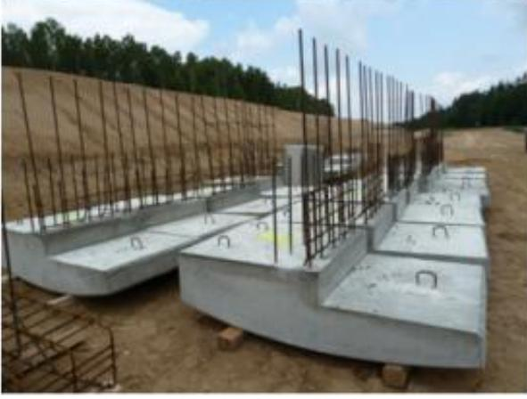
Then prefabricated elements of cornice were placed:
