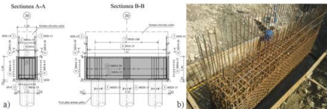
Figure 51 - Foundation slab reinforcement plan (a), Site photo of the foundation slab reinforcement (b)
