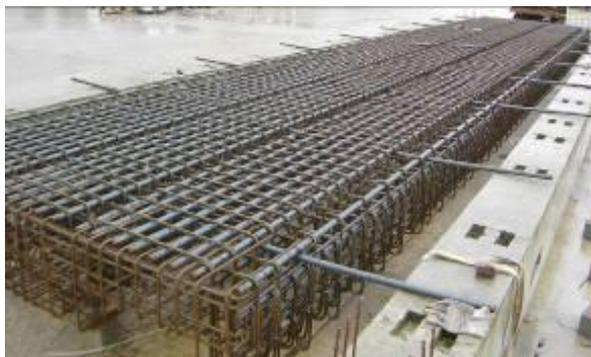
Figure 9 - Reinforcement cage prepared
