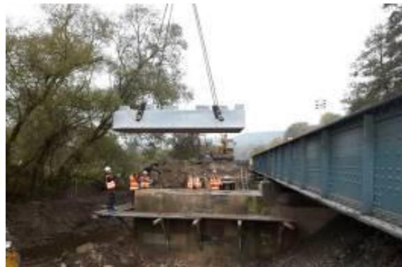
*Figure 23 - Lifting of prefab-benching*
