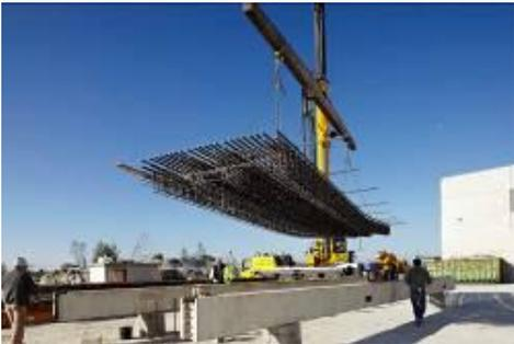
Figure 13 - Lifting of reinforcement-cage
