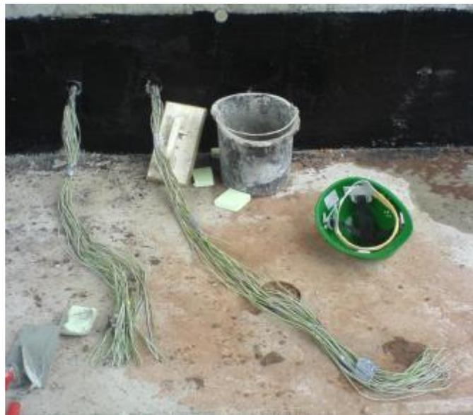
Figure 87 - Measurement wires Leuna, cut-off after installation
