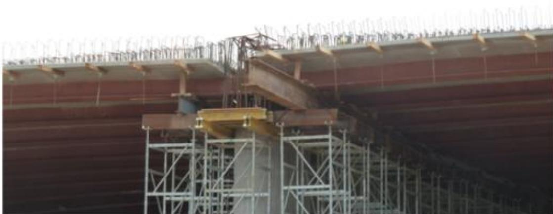
The view from the bottom of the bridge (picture below) presents prefabricated girders of line 2 on temporary supports and realised structure of line 1:
