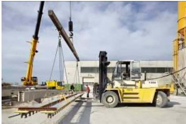
Figure 17 - Transport of external sections
