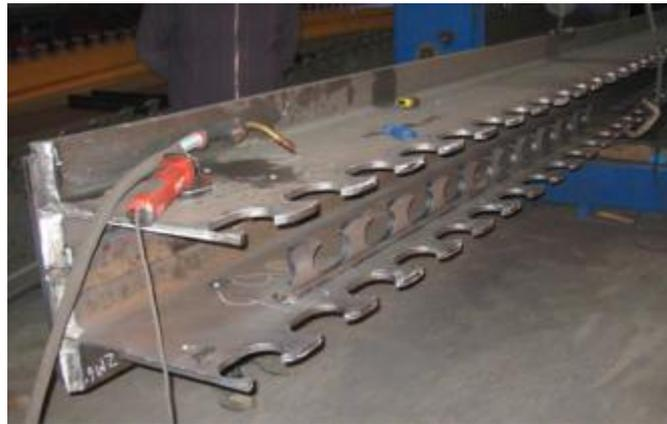
Finally developed formulas for design of composite dowels (after the realisation of PE4, during PRECO+ RFCS project [5]) proved, that PE4 Bridge is safe even without them. But at time of design of bridge we have no formal formulas so we decided to use additional elements.
