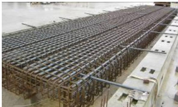
Figure 9 - Reinforcement cage prepared
