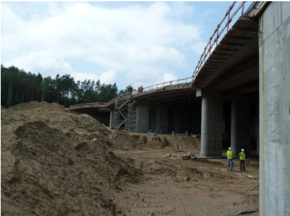
The next steps were to make embankments behind abutments, side concrete elements and soil on the superstructure.
