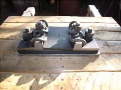
Figure 12 - Rail support before mounting
