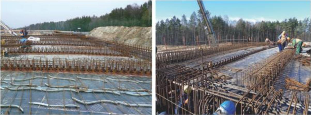
After the prefabricated plates of girders had been casted, intermediate temporary supports were removed (to get the same stage as for prefabricated girders shifted by crane and put in their final position on supports):
