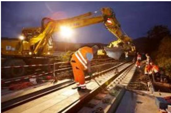
Figure 28 - Assembly of rails
