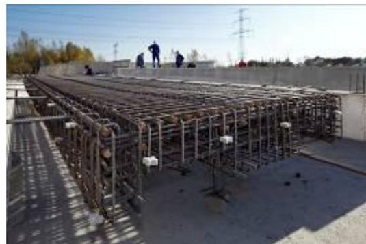
Figure 10 - Reinforcement for first girder
