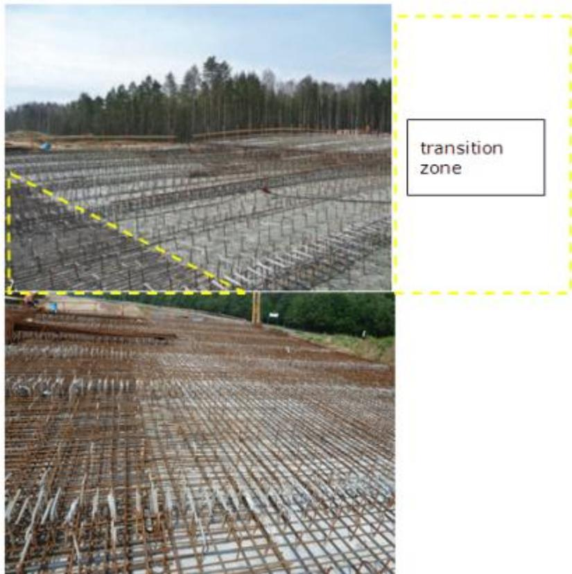
In step 2 additional reinforcement for 5m long transition zone next to supports (stage II of composite section) was implemented.
