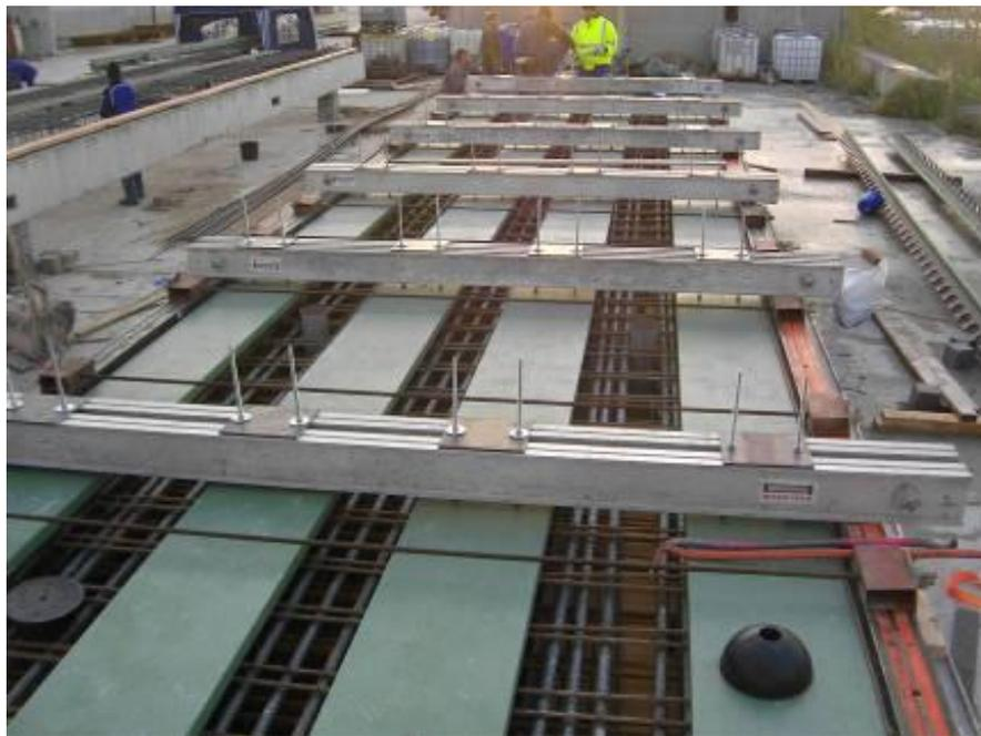
Figure 19 - Formwork prepared with all constructional elements before concreting
