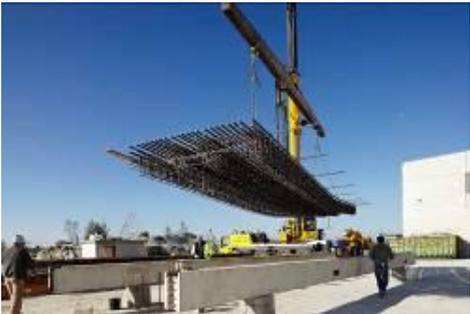
Figure 13 - Lifting of reinforcement-cage
