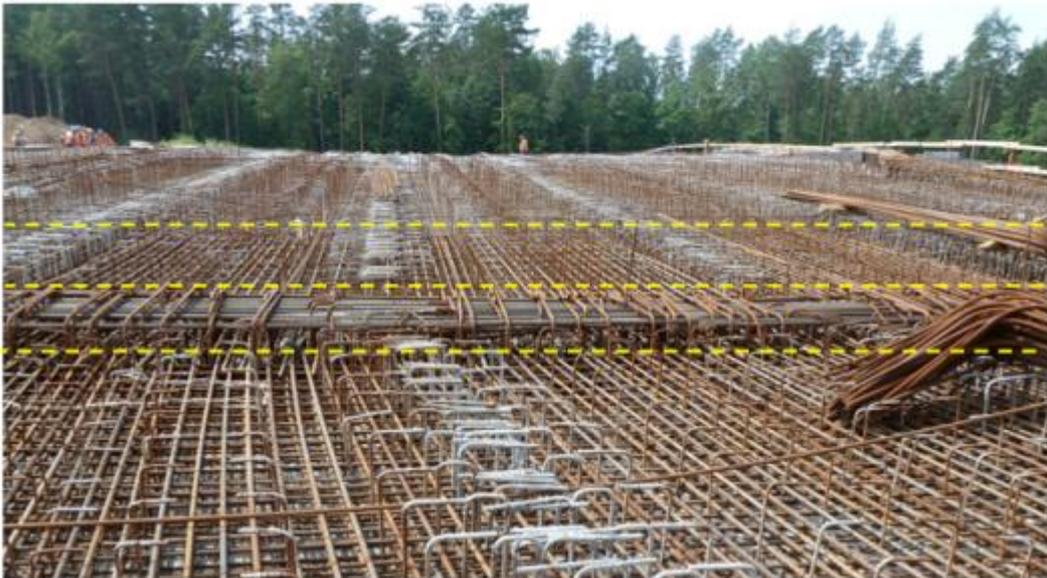
After completion of entire reinforcement of in-situ final slab the transition zones were casted together with crossbeams according to design concept.
