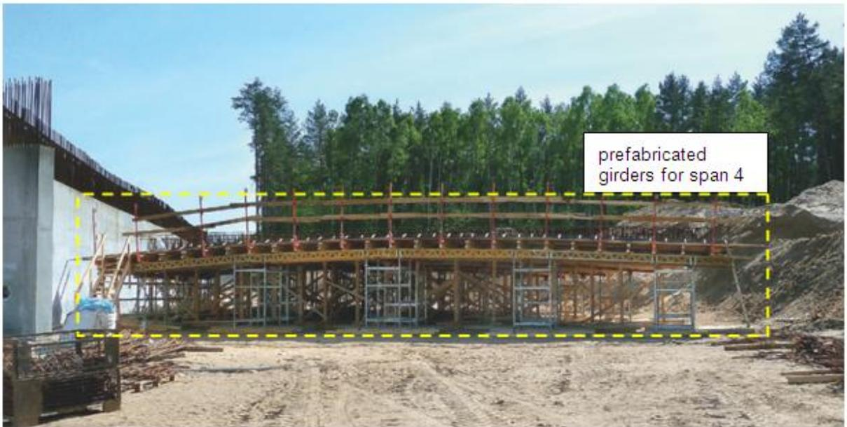
Girders have been realised and they were shifted by crane to their final positions on temporary supports next to pillars and abutments. Temporary supports were necessary to realise scaffolding for crossbeam proper way also.
