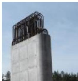
It was very hard to place crossing bars of crossbeam, pillar and prefabricated girder.
