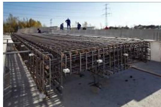
Figure 10 - Reinforcement for first girder
